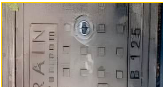
Condition of the socket type keyhole lifting arrangement of THERMODRAIN FRP manhole covers.
